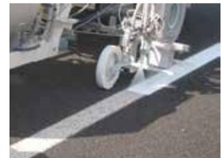
Preco Cryl Spray-Applied Resin 2K can be applied using all conventional application methods with airless and atomiser techniques.
