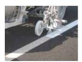
Preco Cryl Spray-Applied Resin 2K can be applied using all conventional application methods with airless and atomiser techniques.
