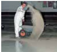
5. The wet coating is sanded down with quartz sand in excess.
