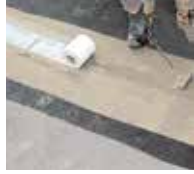
3. ... joints are waterproofed using Triflex ProDetail.
