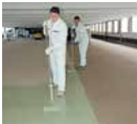
4. Apply the coating Triflex Cryl Finish 209 evenly.
