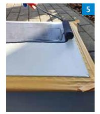
**Sealing:**Seal the fully cured surface with Triflex Cryl Finish 205.
