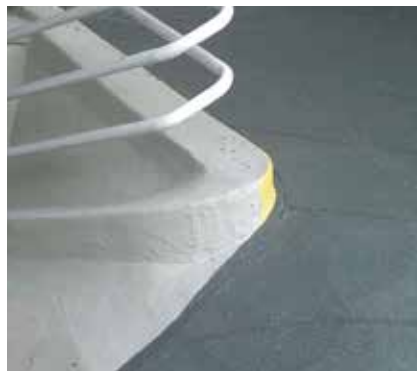
Parking deck – kerb
