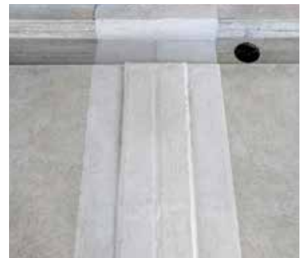
Parking deck – joint
