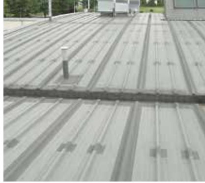
Flat roof – metal roof
