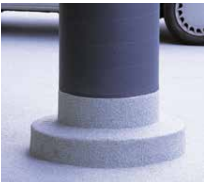
Parking deck – props
