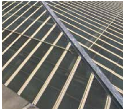
Flat roof – window bars
