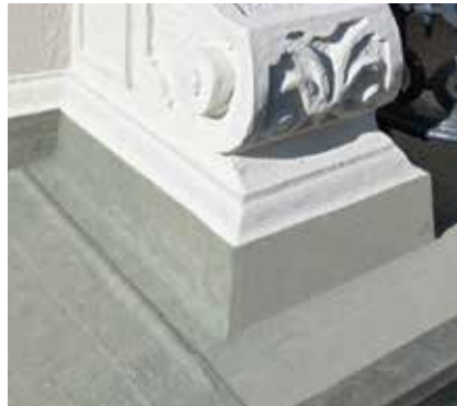
Balcony – wall junction
