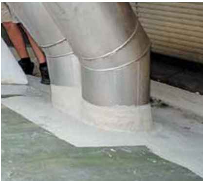
Flat roof – ventilation pipe
