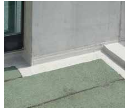
Flat roof – wall junction
