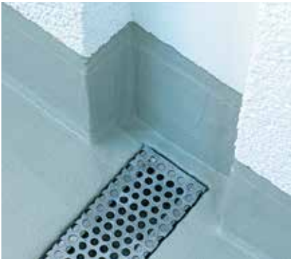
Balcony – gully and gutter
