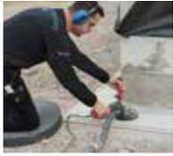
1. For better substrate adhesion, abrade and prepare the concrete.
