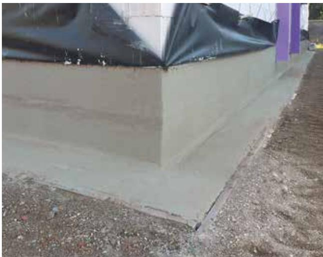
Waterproofing of the structure starts with the foundations being properly and professionally laid. The material used has to meet the challenges of a high water table and rainwater. Only reliable waterproofing of the foundation and base will ensure the durability of a building.
