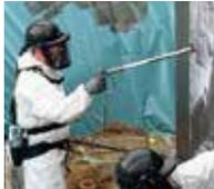
2. ... Triflex SmartTec Sp can be applied using a spray method.
