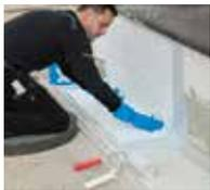
5. ... the Triflex Special Fleece PF is laid, ensuring that there are no air bubbles, and smoothed out with a dry roller ...
