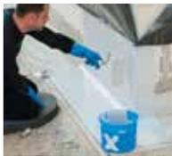
6. ... and a second layer of Triflex SmartTec is applied.
