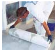
8. Triflex Special Fleece is applied across the entire surface ensuring there are no air bubbles.
