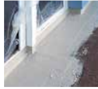
5. A second layer of Triflex ProDetail is applied.
