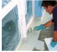
3. First, the details are waterproofed using Triflex ProDetail.
