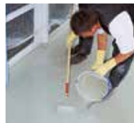
10. The wearing layer of Triflex ProTerra is applied to the surface.
