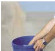
11. For fixed coverings, the wearing layer is dressed with quartz sand.
