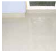
12. Done! Following this, the other covering is applied.
