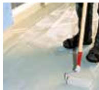
9. A second layer of Triflex ProTerra is applied.
