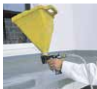
10. ... blow in Triflex Micro Chips.
