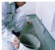
2. Apply Triflex ProDetail to joints.
