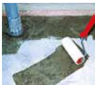
1. Prime wall junction and surface.
