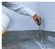
4. ... apply generous coating of Triflex ProDetail.
