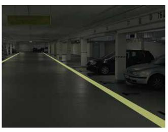
Preco Cryl Cold Plastic 2K NightLine is used as additional safety to supplement existing emergency light systems to indicate escape and rescue routes which are subject to high mechanical loads in staircases, underground car parks, factories, shopping centres, tunnels and so on.
