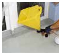
13. ... blow in Triflex Micro Chips.
