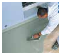
11. ... apply and spread evenly using a notched trowel.
