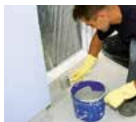
12. Apply the finish Triflex Ceryl Finish 205 and ...
