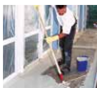
7. Triflex ProTerra is applied generously to the surface.
