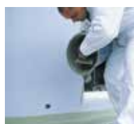
10. The wearing layer: Spread and level out Triflex ProFloor ...
