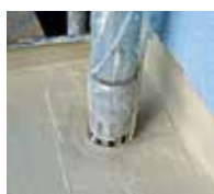
6. The details are completely waterproofed.
