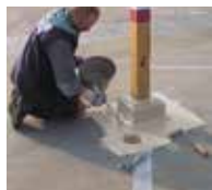
3. First, all details are waterproofed using Triflex ProDetail and ...
