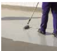
5. Triflex ProPark is applied generously to the surface.
