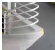
10. ... ramps are additionally coated with Triflex Cryl M 264 or Triflex Cryl M 269.
