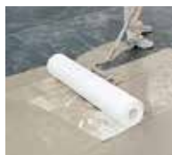
6. Triflex Special Fleece is applied across the entire surface ensuring there are no air bubbles.
