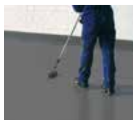
8. Triflex Cryl Finish 209 is applied in the recesses.
