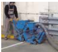
1. Preparation of substrate, e.g. by shot-blasting.
