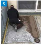
Fill the surfaces between the aligned elevation edges with Triflex CeFix Screed 631 and process while still fresh. Compact the material with gloved hands and a smoothing trowel. Layer thickness from 20-100 mm.
