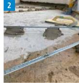
The straightedge is guided along the edges which have already been lightly tightened.
