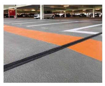
Top decks and parking decks are often large areas that are subject to severe loads and stresses. Expansion joints absorb the movements from subsidence, expansion, vibrations and additional traffic loads. The joints themselves must be reliably sealed for the parking deck waterproofing or coating to provide reliable protection for the concrete substrate.
