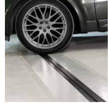
No metals are used in the Triflex ProJoint joint profiles, so they cannot corrode and are resistant to frost and aggressive de-icing salts. The Triflex ProJoint joint profile and the adjacent Triflex multi-storey car park coating have a similar coefficient of thermal expansion. This means that a leak-tight and frictional bond between the materials is guaranteed. Refurbishment intervals are thus extended by years.
