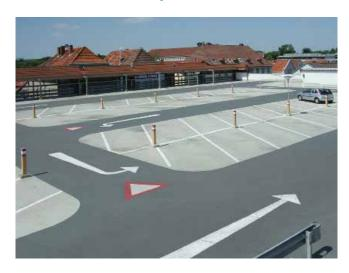
**Triflex ParkLine** is used for marking outdoor parking and set-down areas. The low-solvent, 2-component high-solid paint, which has an epoxy resin base, can be used on asphalt and concrete surfaces. The sprayable Triflex ParkLine offers excellent adhesion, even on substrates with residual moisture. Thanks to the short drying times, the closure times are also very brief.
