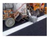
application of profiled markings, an appropriate special unit for conventional cold plastic marking machines is all that is required.
