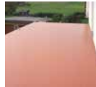
10. Then the Triflex BTS-P waterproofing system is applied.
