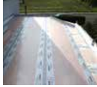
3. ... mark out surface with edging strips.
