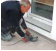
1. Prepare substrate, e.g., by grinding or milling.
