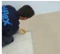
8. ... join with tongue and groove and ...
