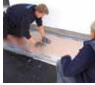
2. Lay vapour barrier and ...
