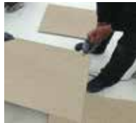
7. Cut the wood-fibre cement boards to size, ...
