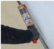
6. Seal edges and seams.
